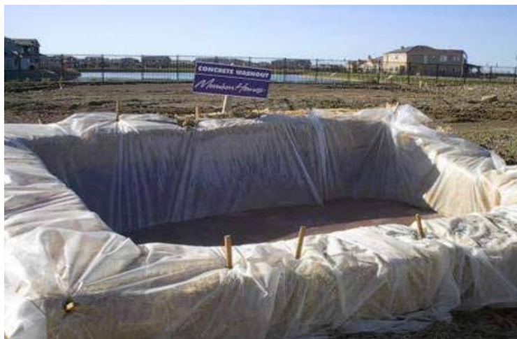
Plate 2.1: Typical Temporary Concrete Washout Area
