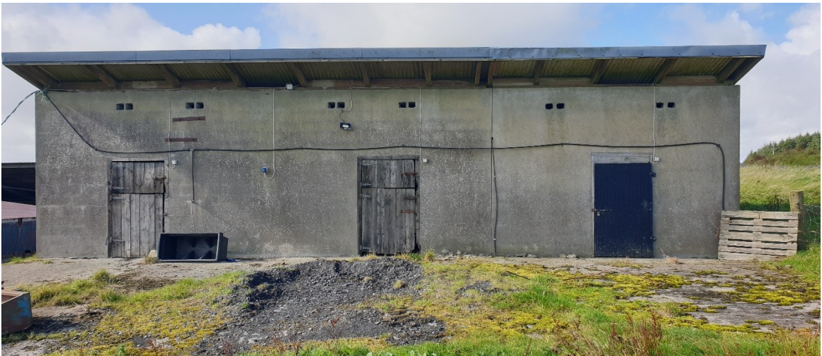
Plate 2.4: Hay Shed for Demolition
